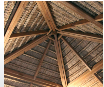
PRE-FABRICATED THATCH ROOF
